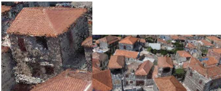
Fig. 10 Parts of the 3D point cloud derived by nadir and oblique images acquired on 25th June 2017, where building damages of grade 4 are clearly identifiable
