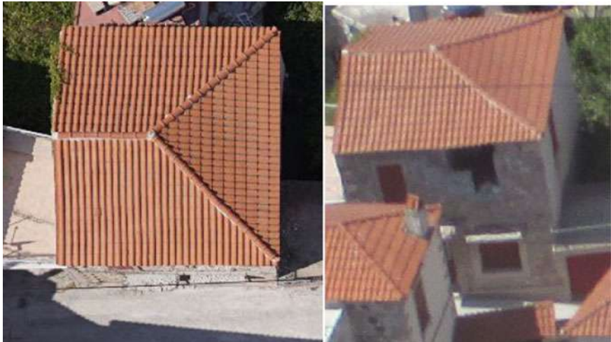
Fig. 9 Part of a nadir (left) and oblique (right) image acquired on 25th June 2017. A serious failure of the top part of a wall is captured only on the oblique image (right)
