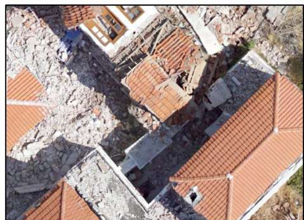
Figure 8. Part of the 25 th July 2017 orthophoto map at a scale of 1:200 which clearly shows damages of grade 3, e.g. dislocation and fall of roof tiles, detachment of the roof from the rest of the structure and fall of gables.
